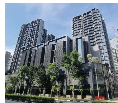
The M Condominium
