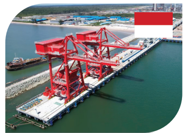
AMI's Aluminium Smelter Jetty, Indonesia
