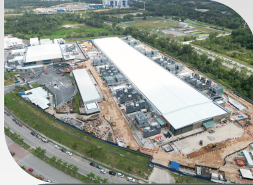
Microsoft Data Center, Selangor
