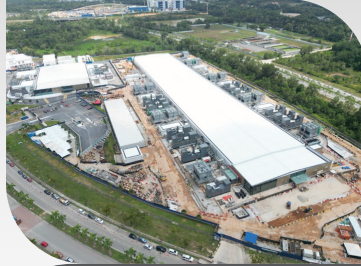
Microsoft Data Center, Selangor
