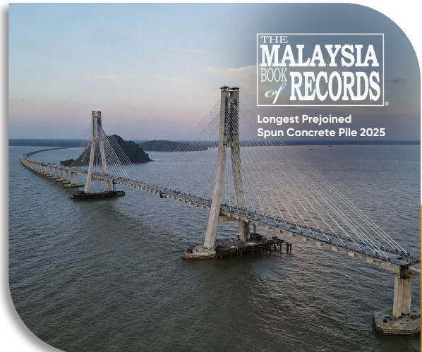
Batang Lupar Bridge, Sarawak
